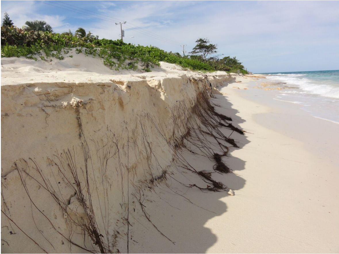
Figure 3.16: Erosion caused by roots and waves at the very Eastern end of Orange Hill Beach (Photo POLZIN, February 2016)
