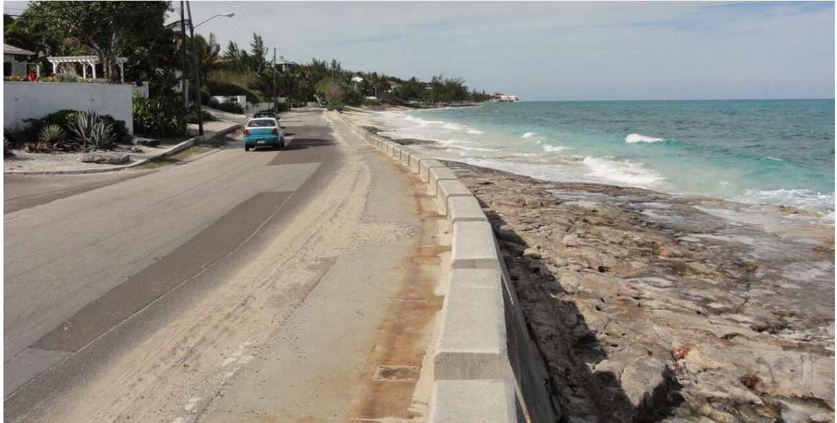
Figure 3.1: Seawall at the corner Bahama West Drive and West Bay Street (Photo POLZIN, February 2016)
