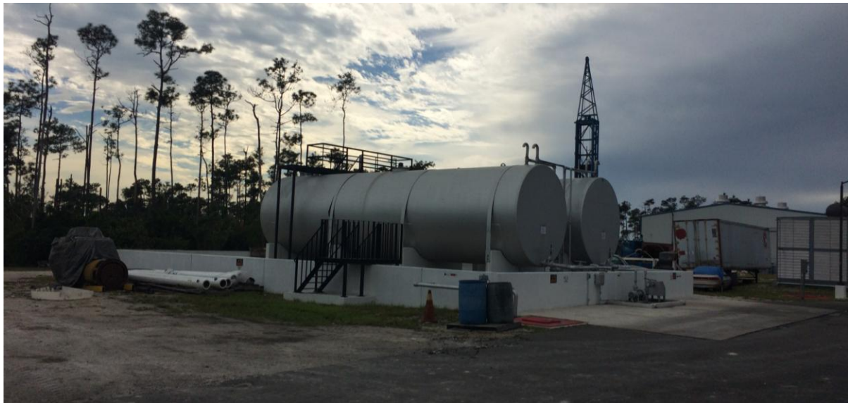
Figure 4.5: Diesel reservoir Blue Hills (Photo Stolle, February 2016).
