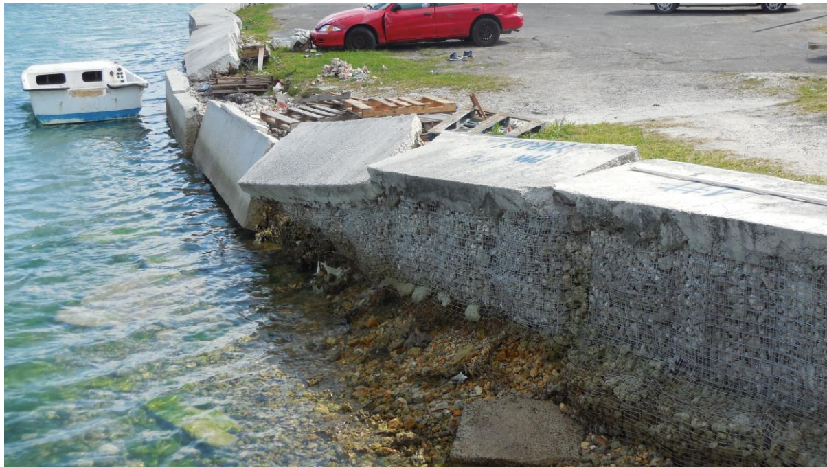
Figure 3.5: An intact and a damaged gabion next to the Arawak Cay Bridge (Photo MICHAELIS, February 2016)
