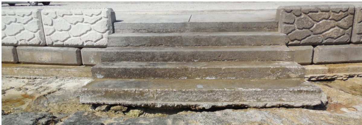
Figure 3.7: A seawall and stairs with undercutting at Eastern Point (Photo MICHAELIS, 2016)
