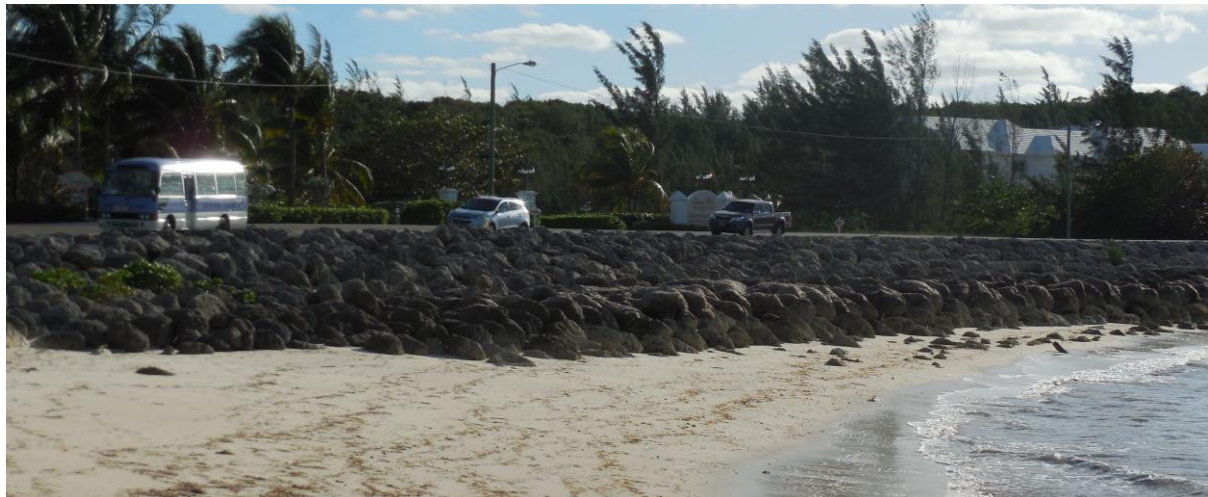
Figure 3.13: Revetment at Rock Point to protect the street from further destruction and erosion
