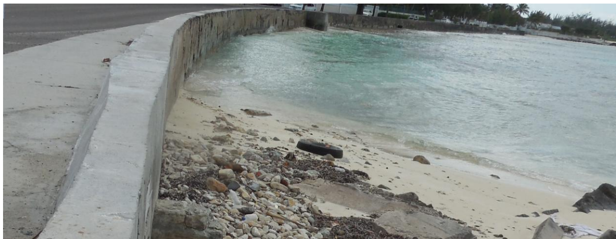
Figure 3.11: A broken seawall at Brown's Point (Photo MICHAELIS, February 2016)
