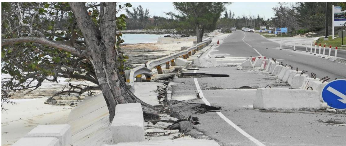
Figure 3.20: Destructive impact of erosion at Caves Point West Bay Street, New Providence (Photo: Neil Sealey, 2013)
