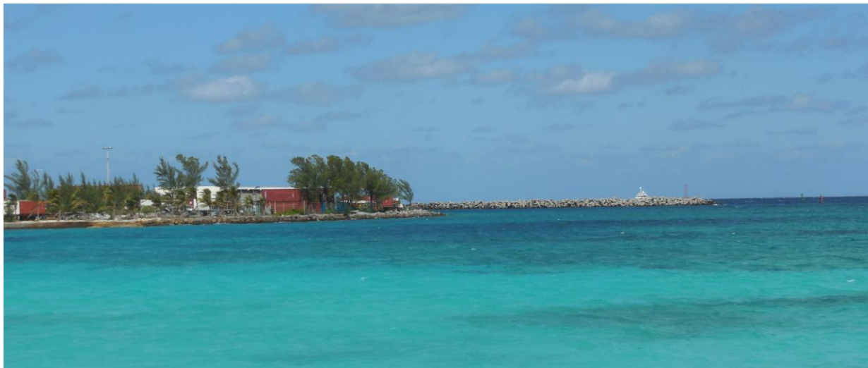
Figure 3.9: Casuarinas on the left and tetrapods on the right in front of Arawak Cay (Photo MICHAELIS, 2016)
