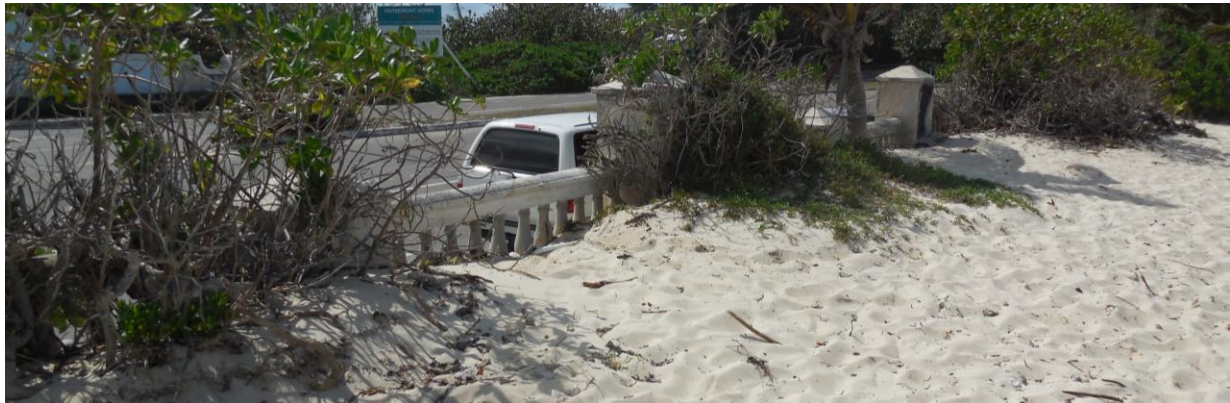
Figure 3.12: Sand stopped by the wall at Sandyport Beach (Photo MICHAELIS, February 2016)
