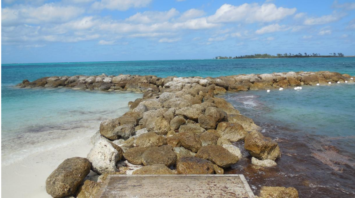
Figure 3.4: Groins at Saunder's Beach (Photo MICHAELIS, February 2016)
