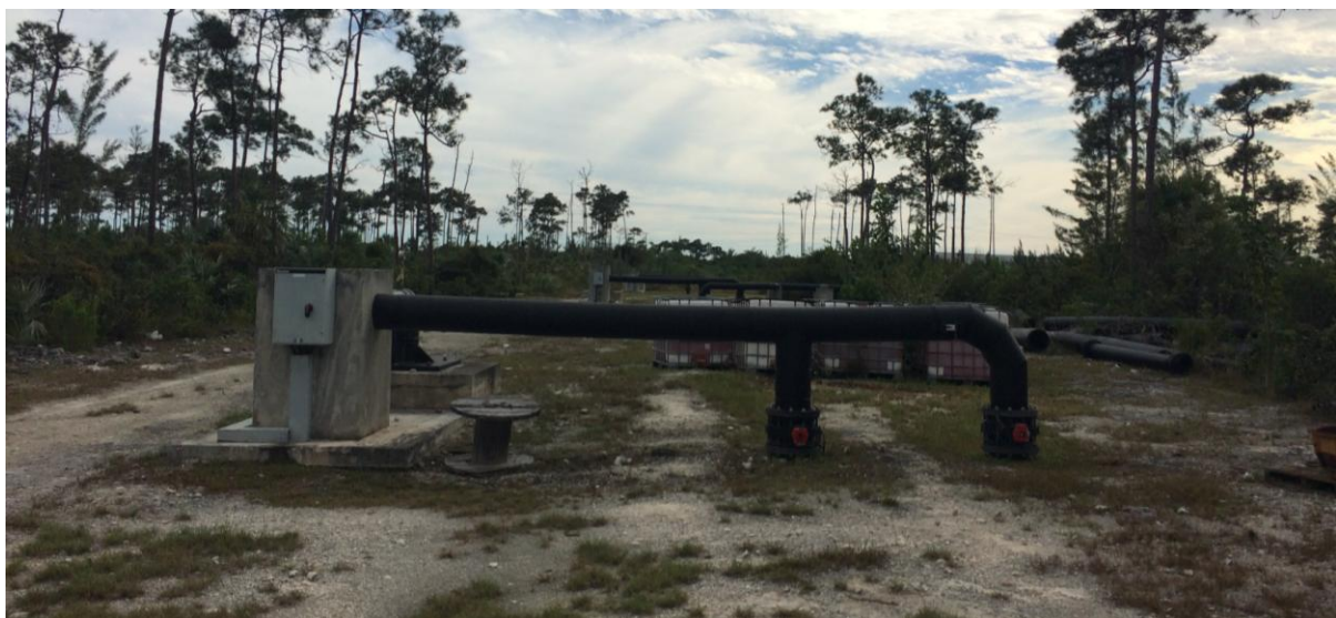
Figure 4.4: Extraction well Blue Hills (Photo Stolle, February 2016)
