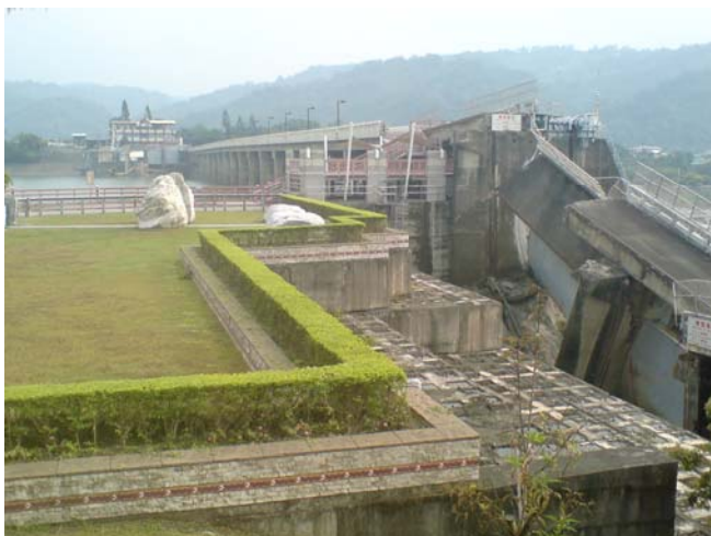
Picture 1: The damaged Shih – kang dam (photo: L. Busch)
