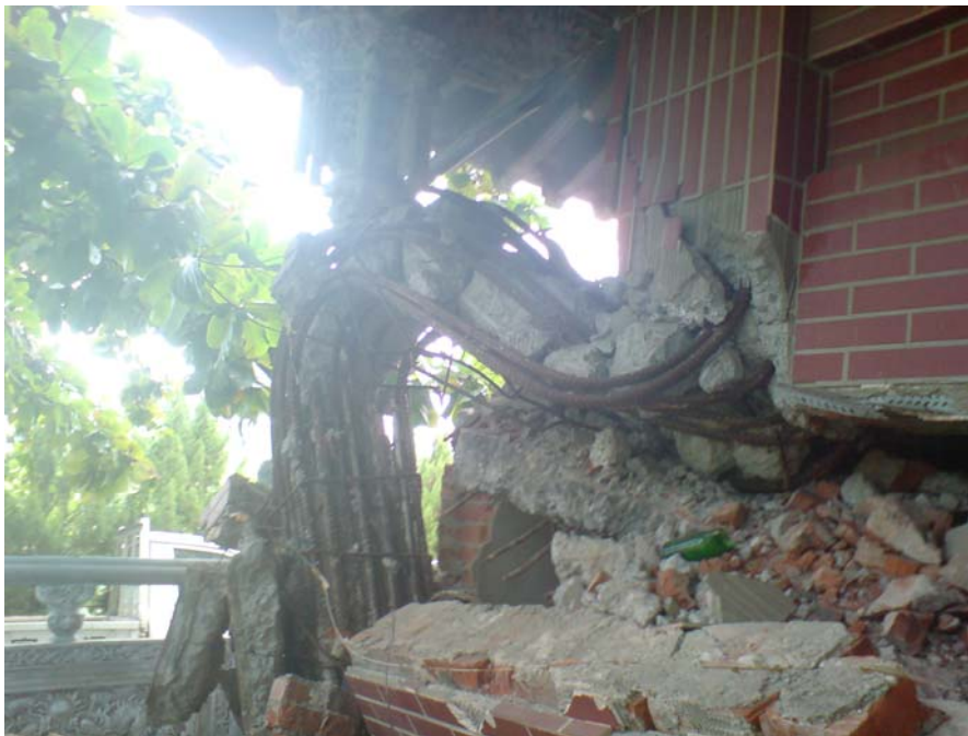
Picture 3: Compressed stanchion of Wuchang Palace (photo: L. Busch)
